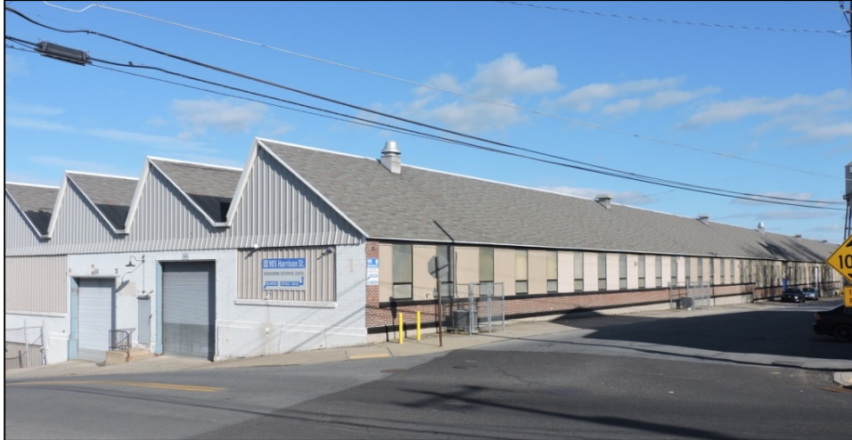
Portion of the repurposed Mack Truck plant in South Allentown
