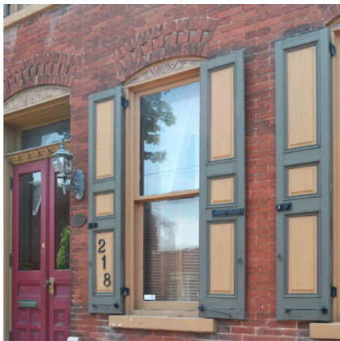
Examples of appropriate paneled wood shutters / blinds.
