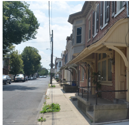
"Allentown" porch roof
