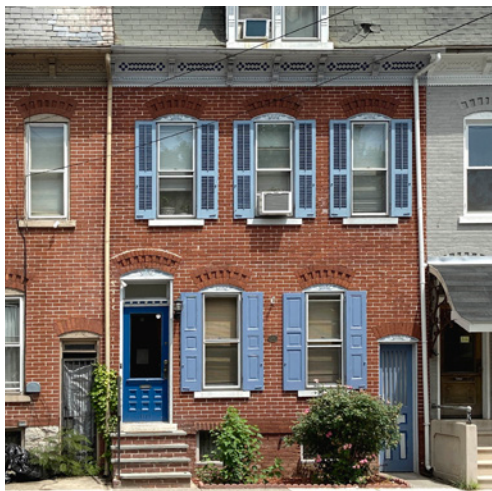
Example of a construction that incorporates blind and movable louvers shutters into the facade
