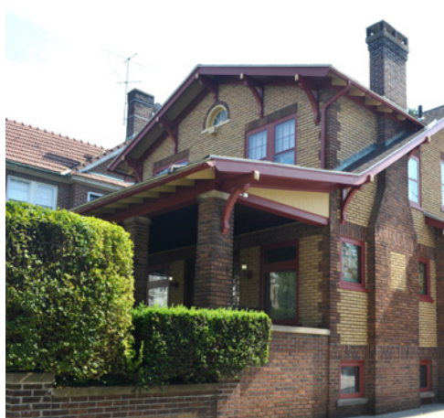
Chimneys that retain original details and are unified with the architectural style of the building should be preserved.
