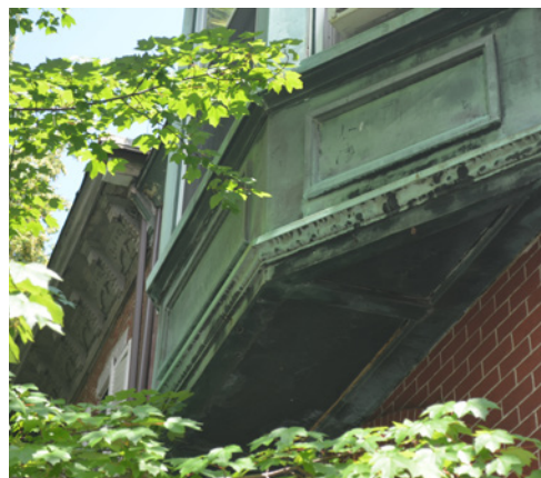
Copper cladding at bay window.
