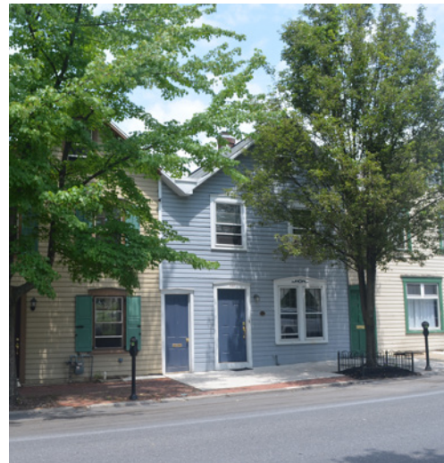
Examples of wood clapboard facades.
