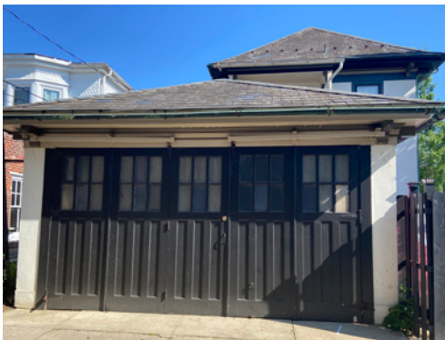
Example of an accessory structure with the same roof type as the main building and distinctive highly-visible doors.
