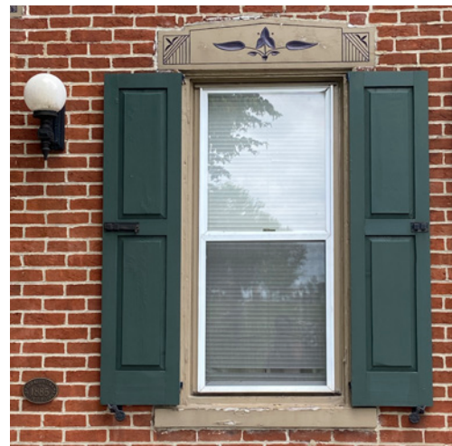
Examples of appropriate paneled wood shutters blinds.
