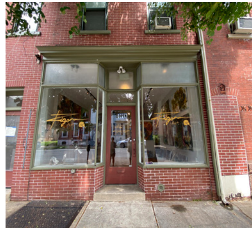
Wood storefront with recessed entrance and transom windows
