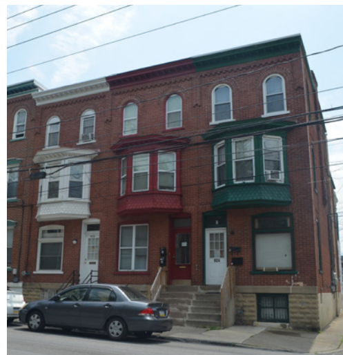
Typical brick masonry construction
