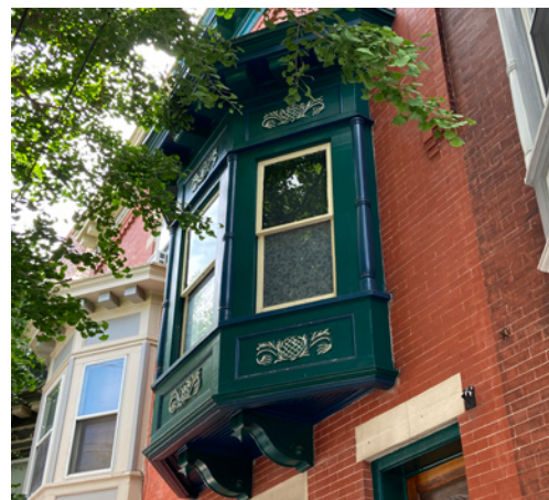
1/1 double-hung wood windows at a bay window.
