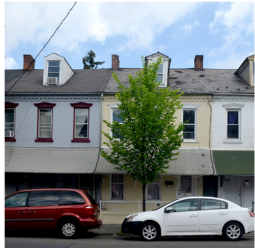
Ridge chimneys that are visible at the shared roof ridge of attached rowhouses contribute to the rhythm of the street.
