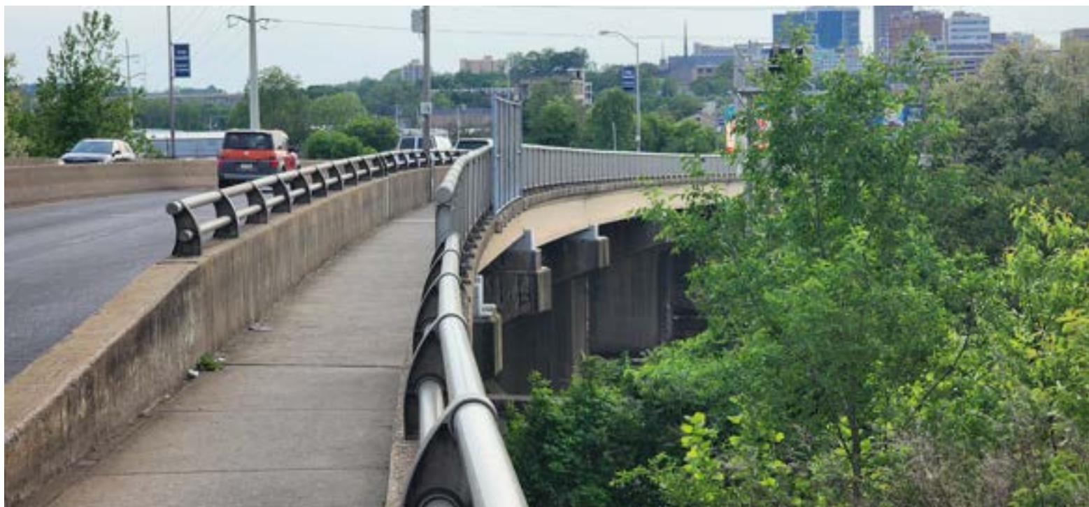
Hamilton Street Bridge over the Lehigh River
