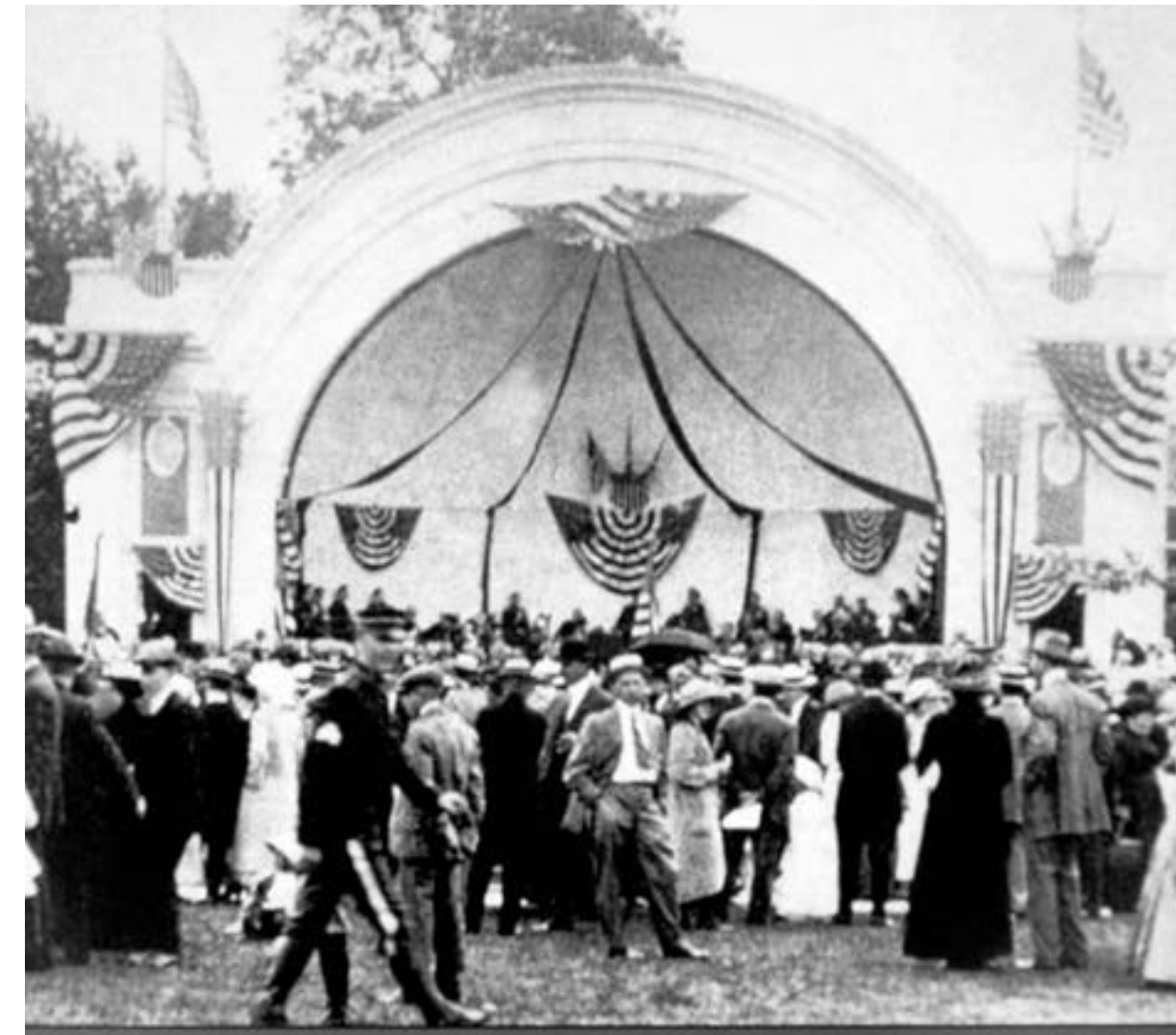
Above: 1911 photo of the shell at West Park, the first park in Allentown
