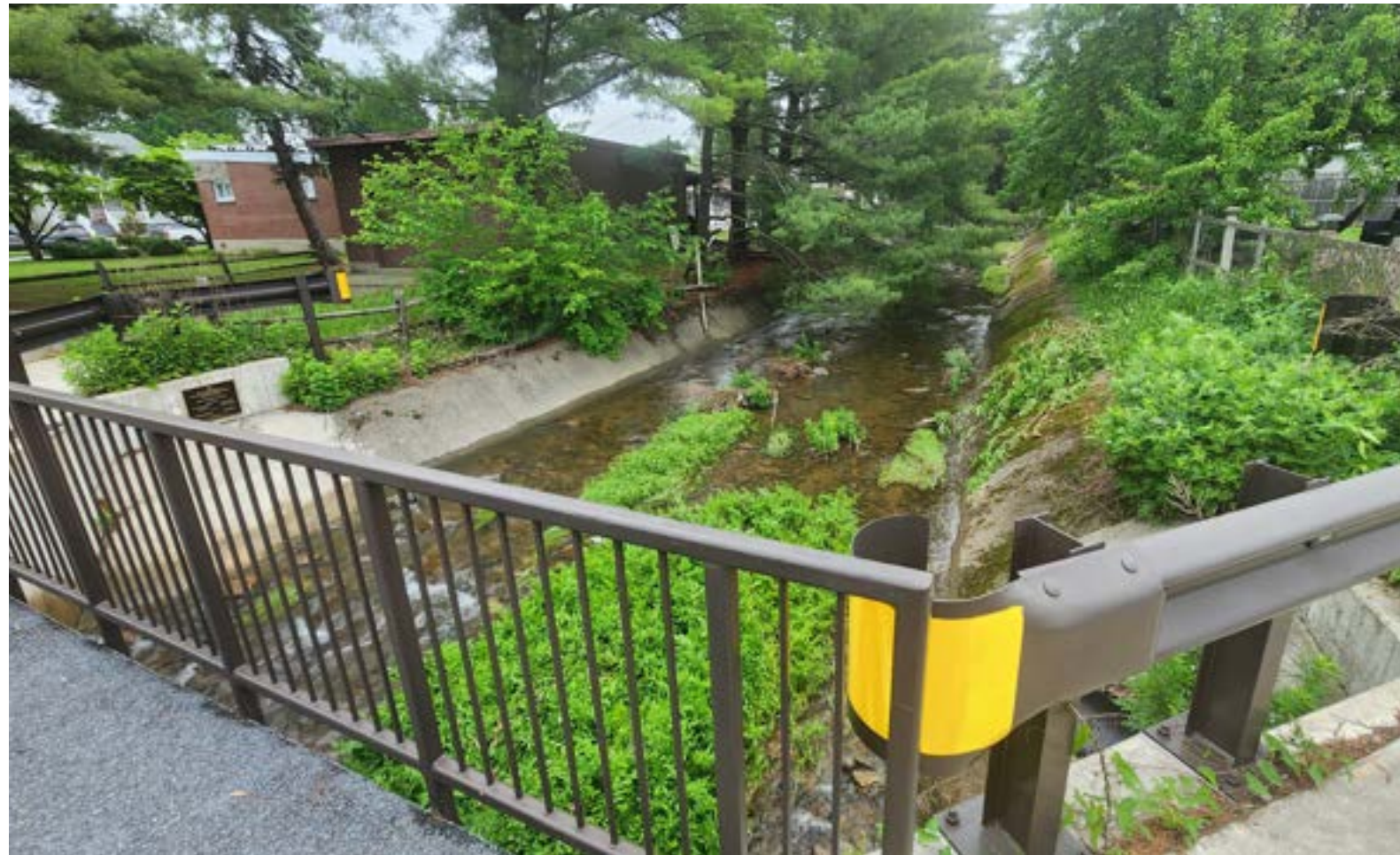
Trout Creek is forced through man-made infrastructure.
