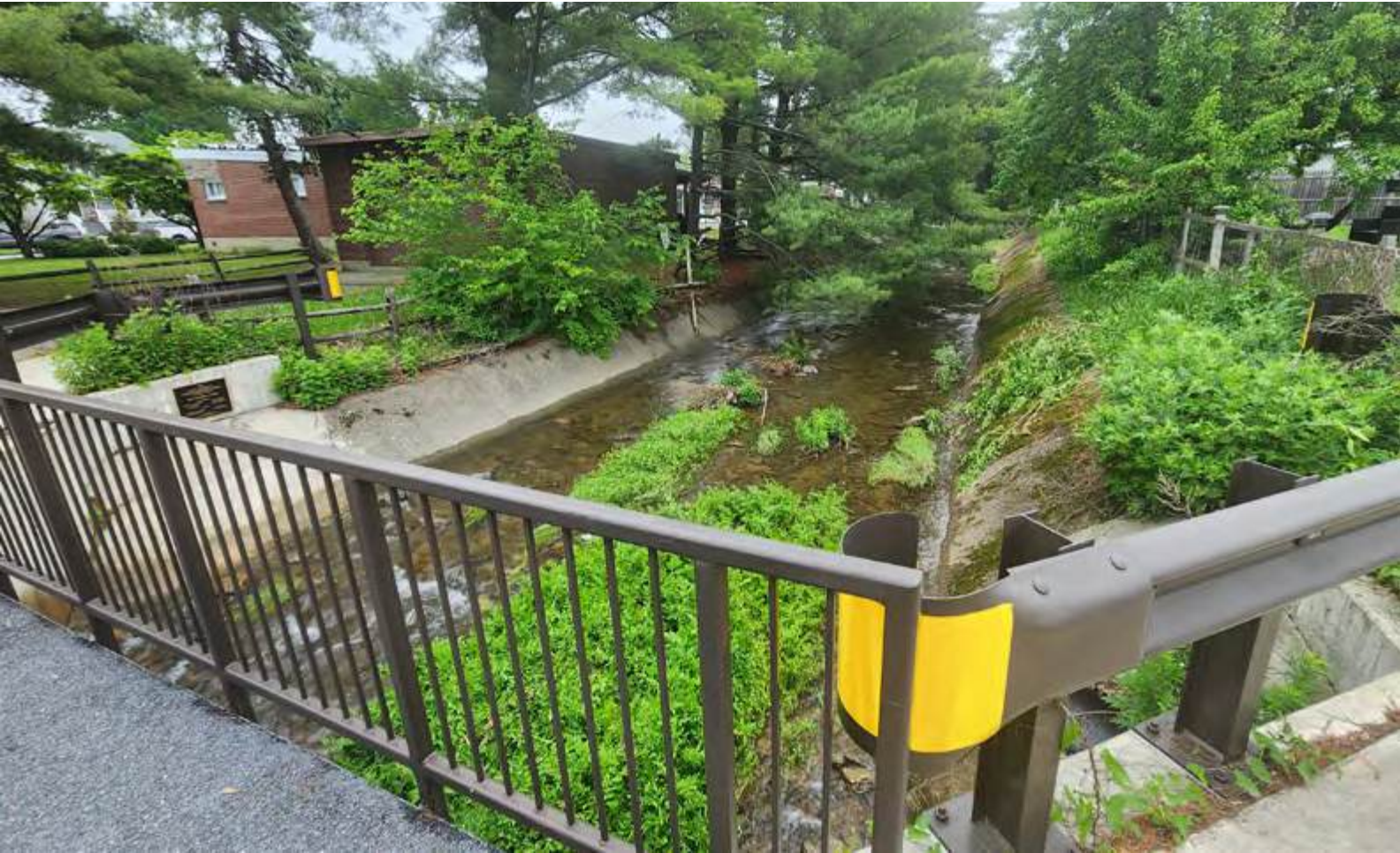
Trout Creek is forced through man-made infrastructure.
