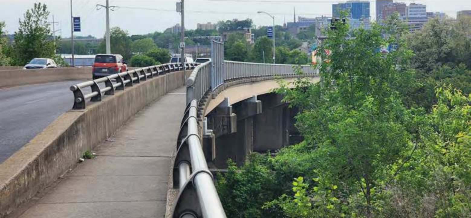
Hamilton Street Bridge over the Lehigh River
