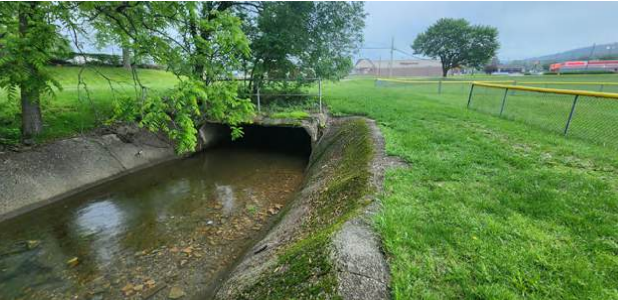
Channelized streams and having lawn up to the edges can create issues with waterways such as introduction of non-point pollutants and flooding when the floodplain has been removed.
