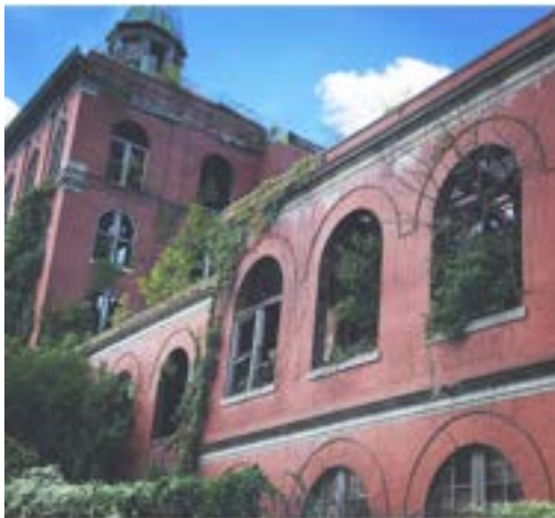
Example of potential adaptive reuse (former Neuweiler Brewery site)
