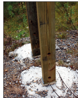
Concrete Foundations with Wood Post Breakaway Feature
