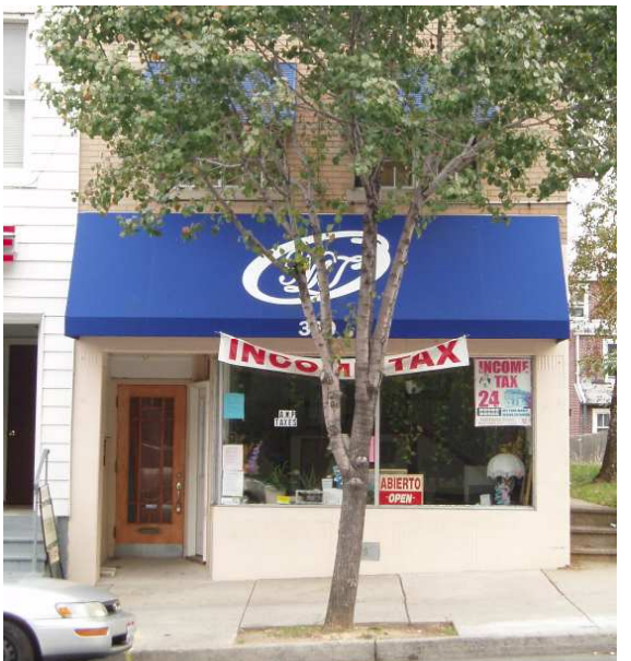
Inappropriate Awning Scale
