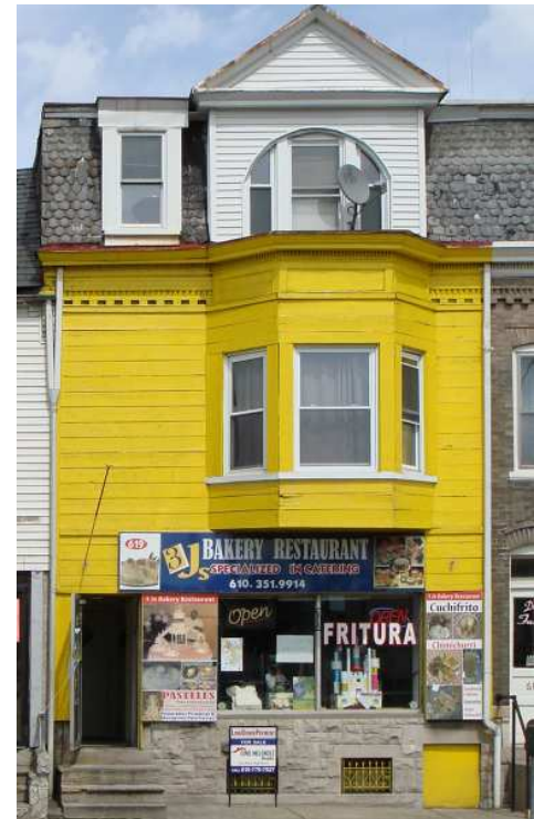
Inappropriate Color & Paint Scheme
