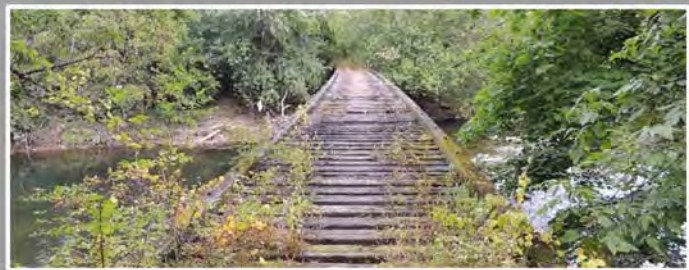
Bridge over Little Lehigh Creek Proposed for Reuse
