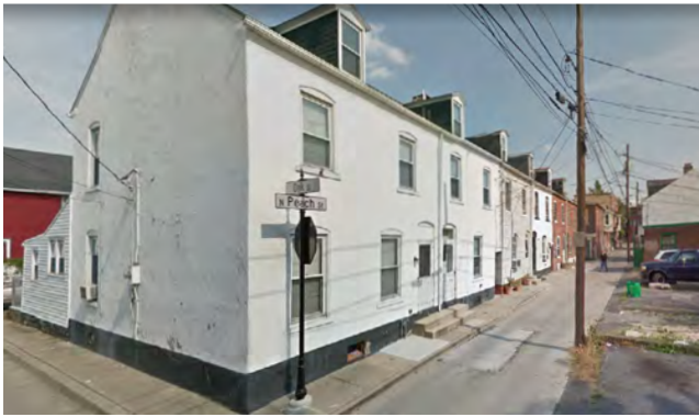
Typical Lane Rowhouses
