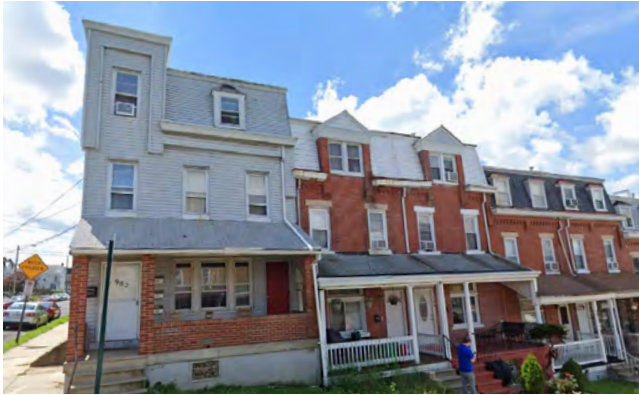
Stacked Units on End of Building
